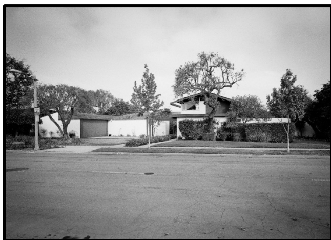
Photograph 13. Hafley House, Long Beach, Los Angeles County, California.
