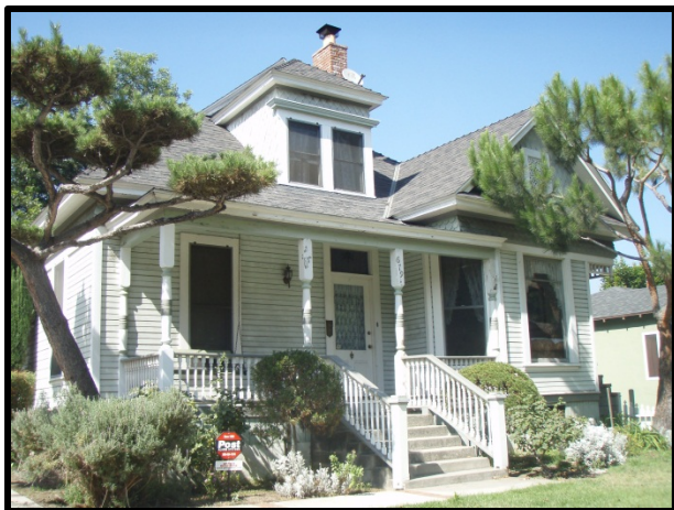
Photograph 23. Friend Lacey House, Pasadena, Los Angeles County, California.
