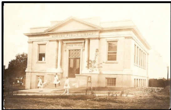
Photograph 37. Auburn Public Library, Auburn, Placer County, California.
