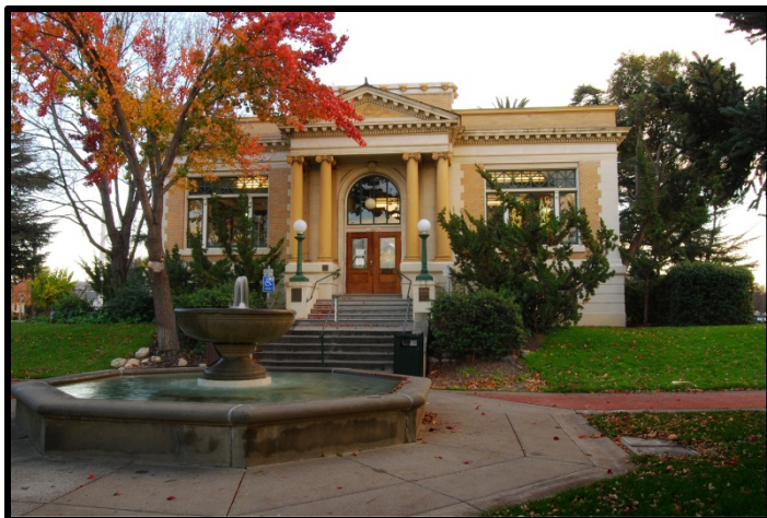
Photograph 7. Livermore Carnegie Library, Livermore, Alameda County, California.
