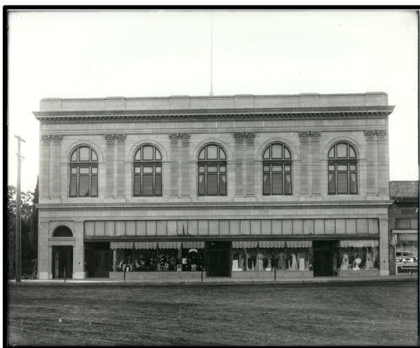
Photograph 36. Auburn Masonic Temple, Auburn, Placer County, California.
