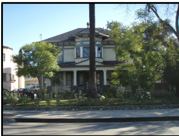
Photograph 26. Raymond-Summit Historic District, Pasadena, Los Angeles County, California.
