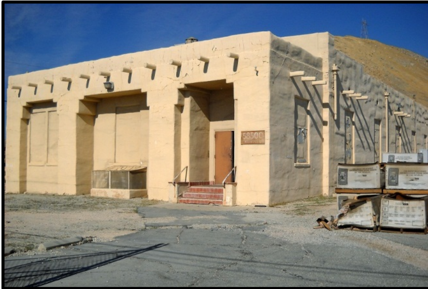
Photograph 58. AT&T Whitewater Repeater Station, Riverside, Riverside County, California.
