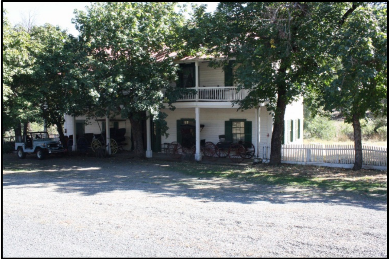
Photograph 54. Forest House, Yreka, Siskiyou County, California.
