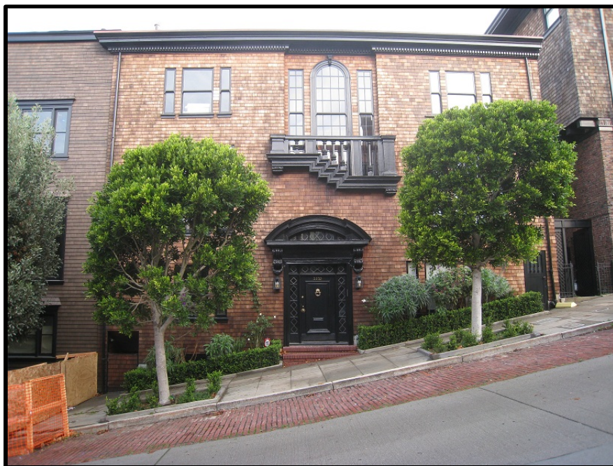
Photograph 51. Julian Waybur House, San Francisco, San Francisco County, California.
