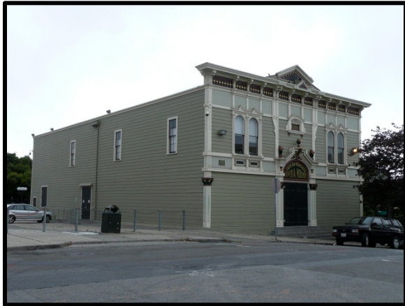
Photograph 50. South San Francisco Opera House, San Francisco, San Francisco County, California.
