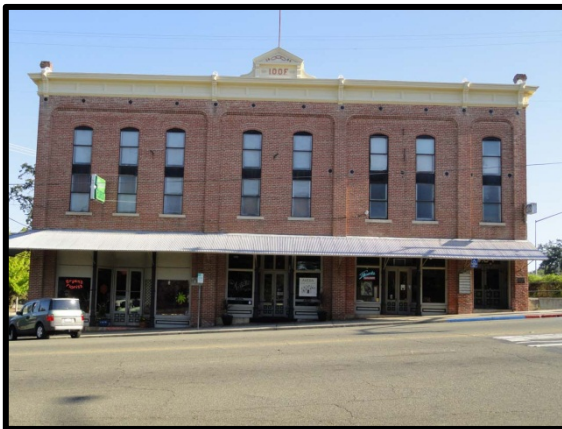
Photograph 35. Auburn IOOF Hall, Auburn, Placer County, California.
